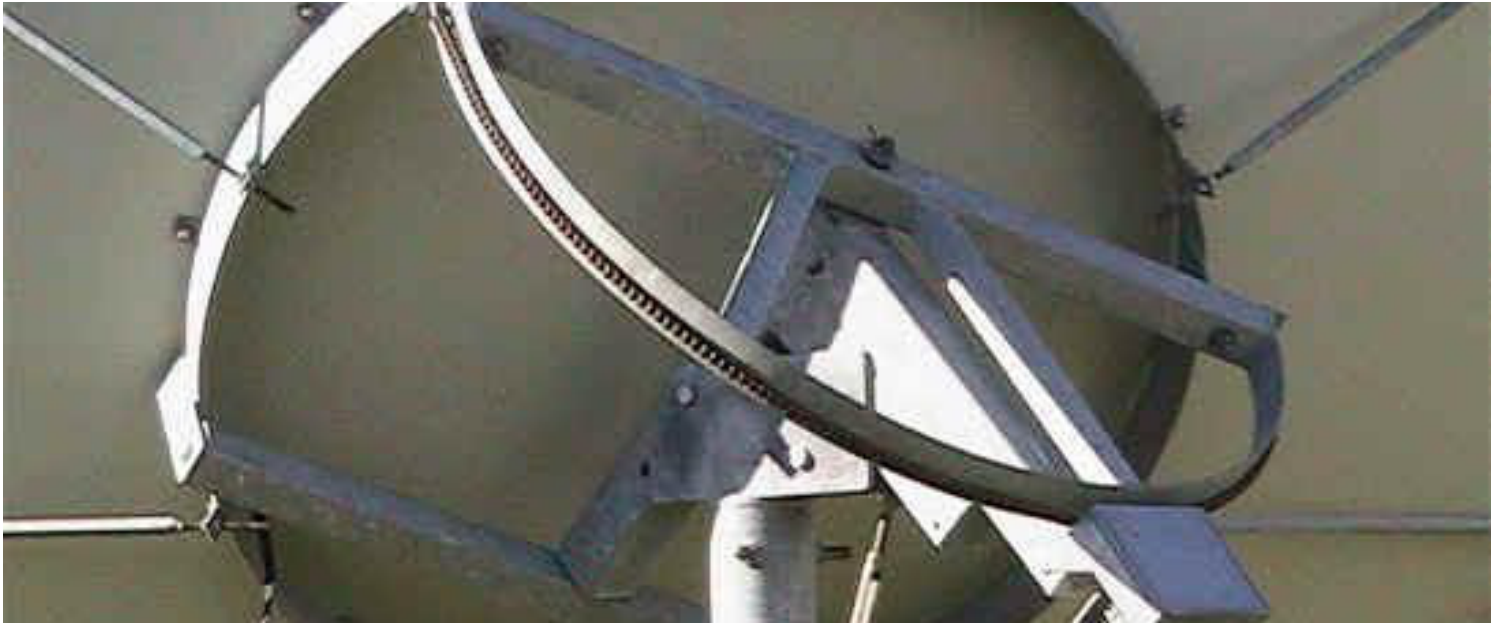
Rear view of a solid multi-panel antenna with a true D-ring chain drive horizon-to-horizon motor, made by DH Satellite in Wisconsin. It's available in sectional panel design for more efficient shipping, in sizes of 3.0, 3.7, 4.2, 4.5 and 5.0 meters. (Courtesy: DH Satellite)
