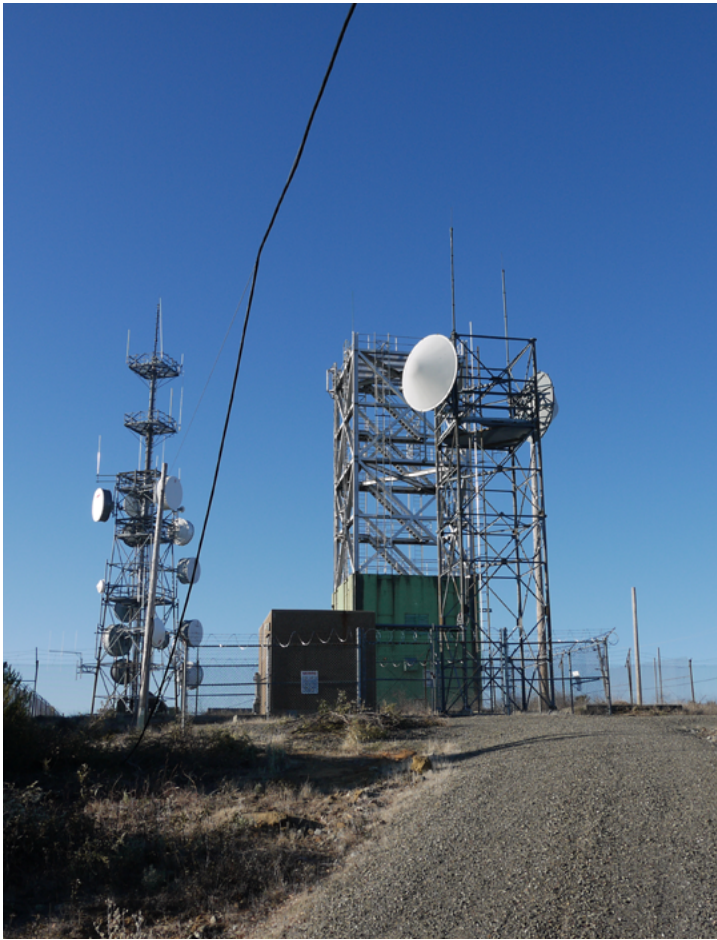
An FAA radio site linked with microwave dishes (courtesy the authors collection)
