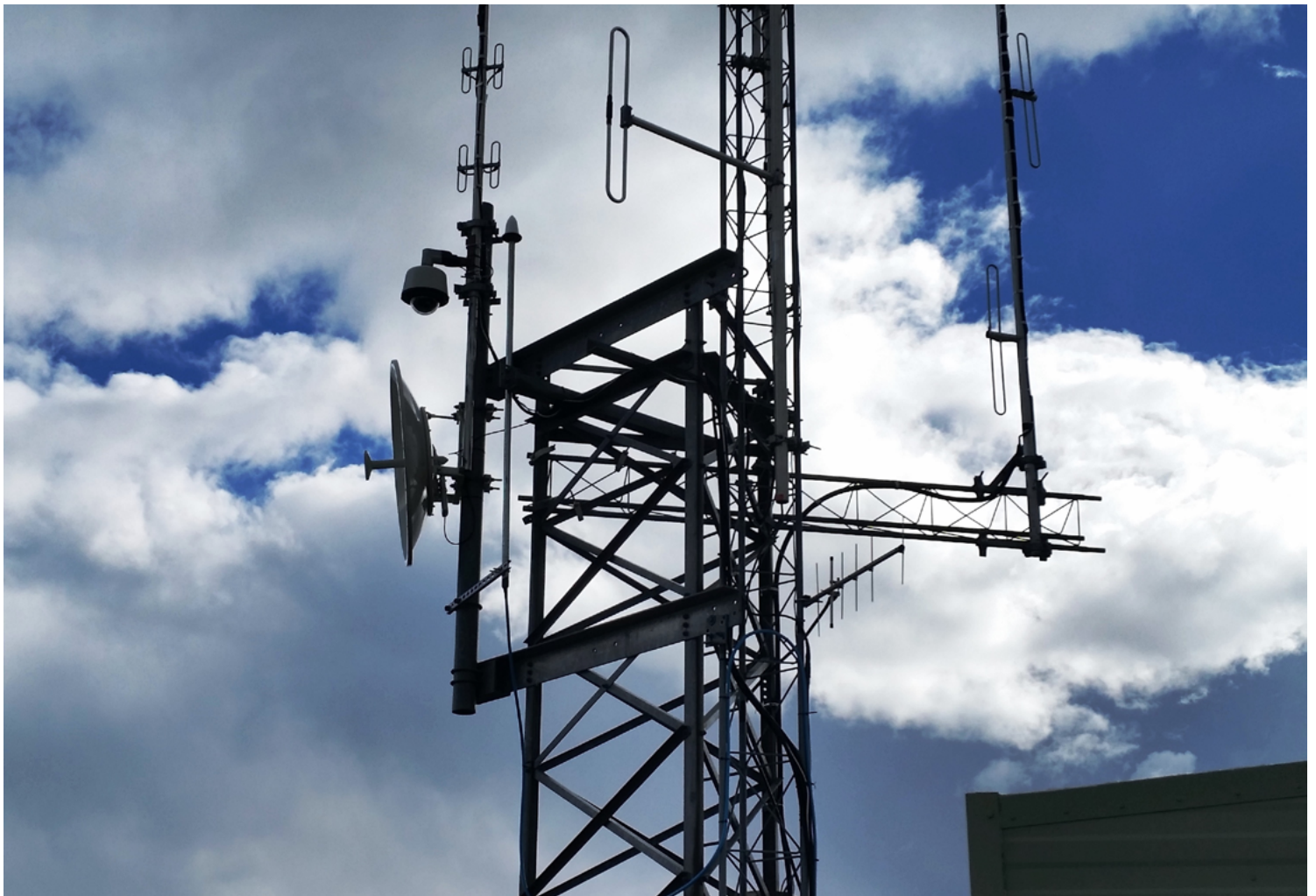
RMHAM microwave relay on Methodist Peak at 11,700 feet. (Photo by Jeff Carrier K0JSC)
