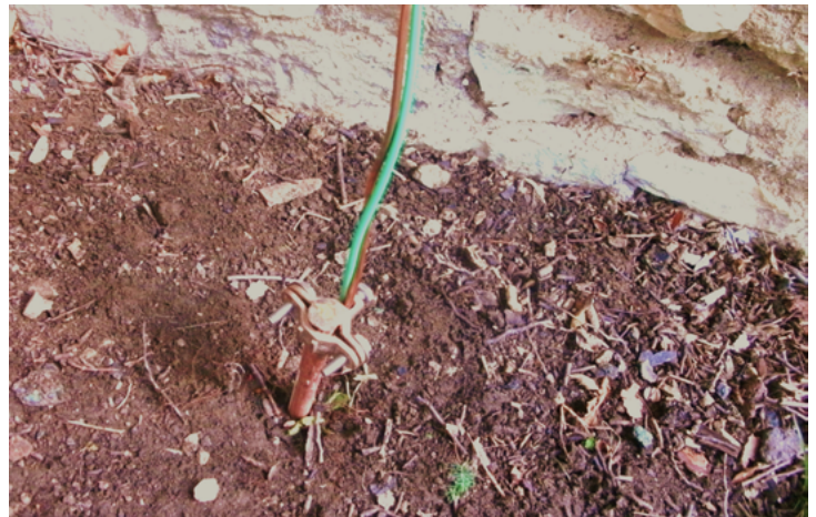
Safety ground at my station. NOT a valid RF ground. (Photo by author)
