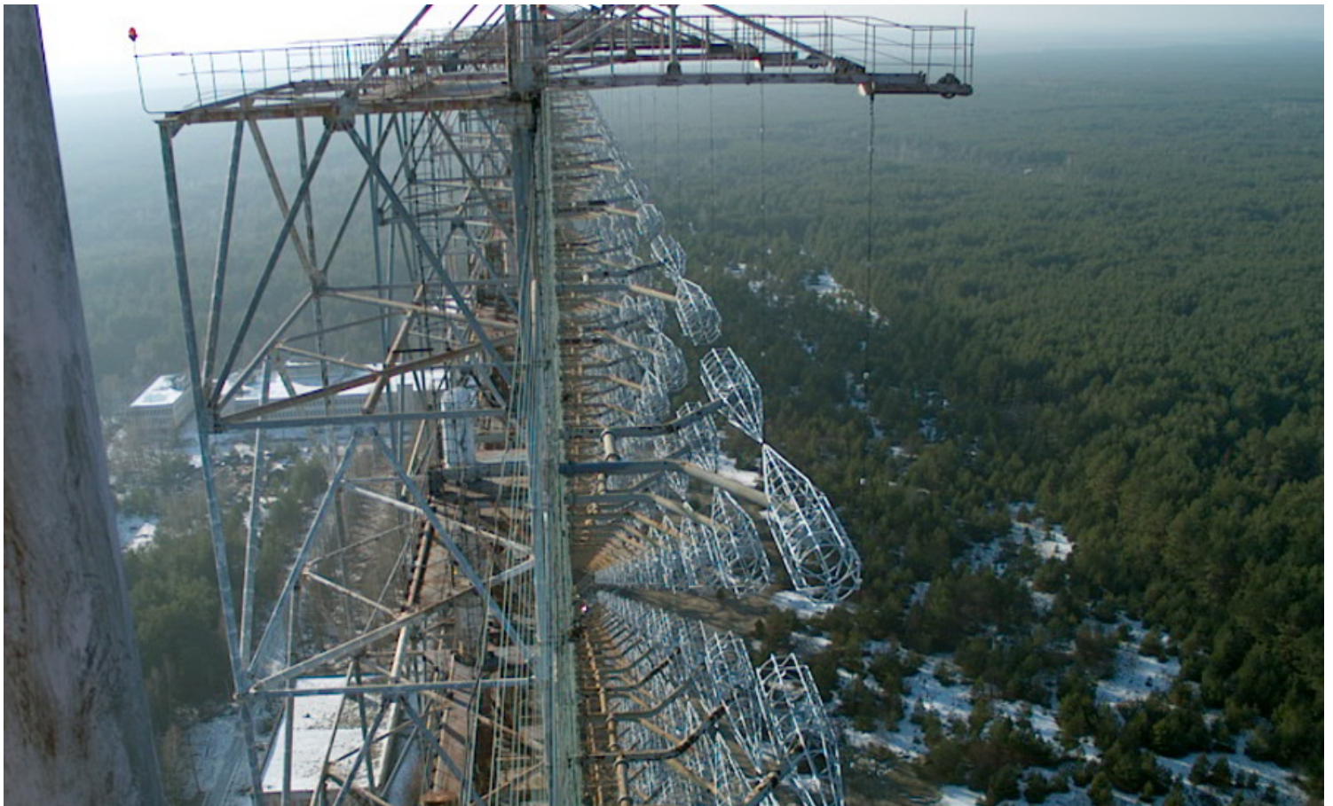
Duga-1 array within the Chernobyl Exclusion Zone. The array of pairs of cylindrical/conical cages on the right are the driven elements, fed at the facing points with a form of ladder line suspended from stand-off platforms at top right. A backplane axial reflector of small wires can just be seen left of center, most clearly at the bottom of the image. (By Necator - the English language Wikipedia (log), Public Domain, https://commons.wikimedia.org/w/index.php?curid=4870433 )
