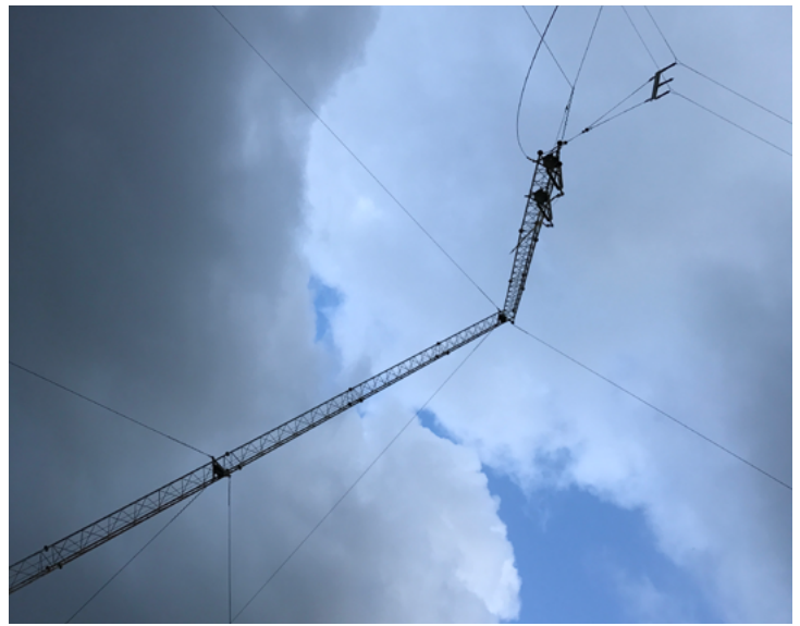
Left: WRMI transmitter building prior to hurricane Irma's arrival. Right: Snapped antenna support tower. (Courtesy: Jeff White, WRMI)
