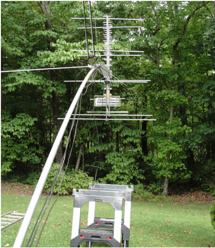
Looking down the flexing mast, just before the splice broke, but the safety rope kept the entire project from crashing to the ground. (KS4ZR photo)
