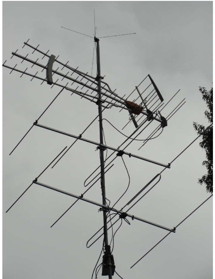
Actually not a black and white photo. Looking up into a dreary overcast day, all four antennas on the mast with rotator in place. (KS4ZR photo)
