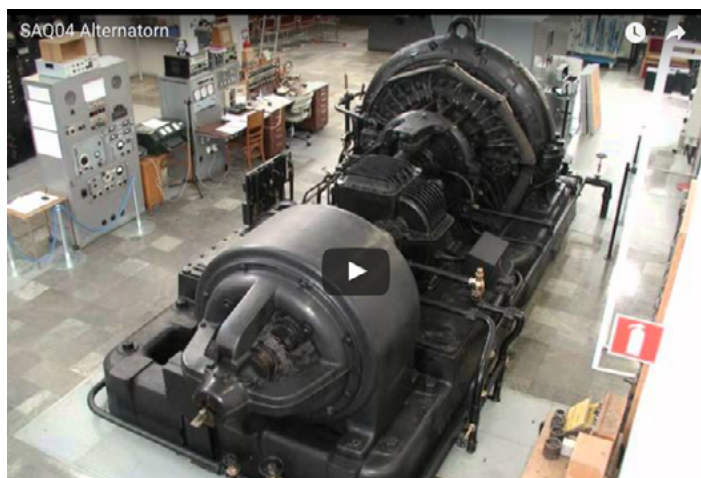
The Alexanderson transmitter set consists of three parts: the driving motor, a gear drive and the high frequency generator, commonly called the alternator. They are assembled on a solid base of steel. The weight of the complete transmitter set is about 50 tons. (Screen shot from a YouTube video of the transmitter courtesy: The Alexander Association. http://alexander.n.se/the-radio-station-saq-grimeton/the-alexanderson-transmitter/?lang=en )
