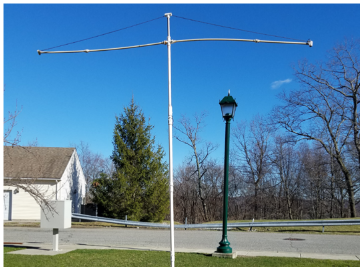
The author's 6-meter antenna work in progress. (N6CL photo)
