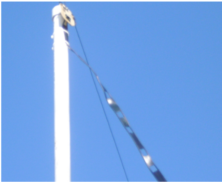
Common “windowed” line, feeding a big dipole. (Author’s photo)
